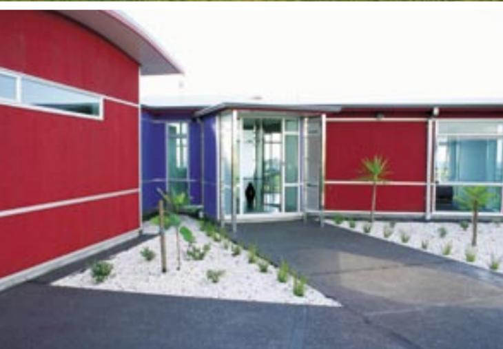
The stylishly curved roof is created with curved longrun steel roofing in 'Habitats Metallic Silver' and painted with 'Colorcote ZRX'. The exterior cladding is Shadowclad texture and plywood.
